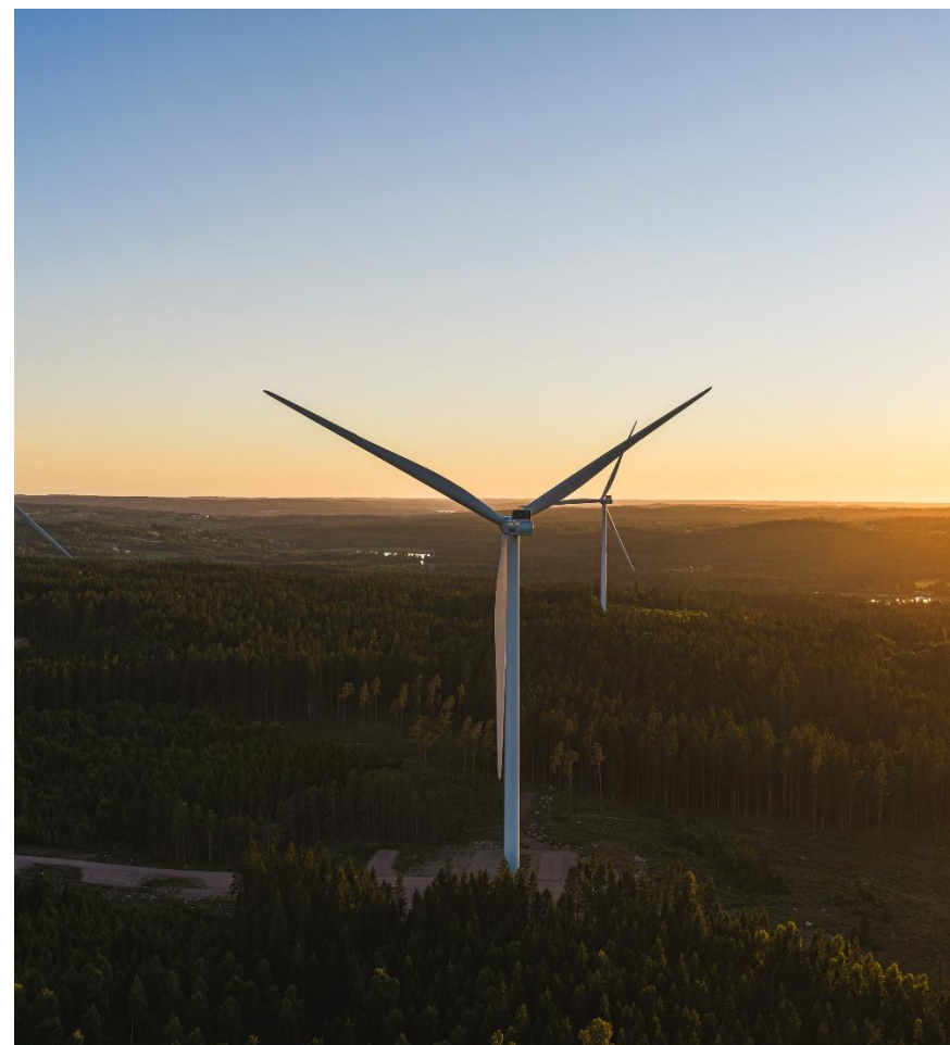
The Dällebo wind park in Ulricehamn Municipality comprises four turbines with a total capacity of 18 MW. On behalf of the owner Mirova, Eolus is now developing battery storage for Dällebo as well as the Fågelås and Boarp wind parks.
